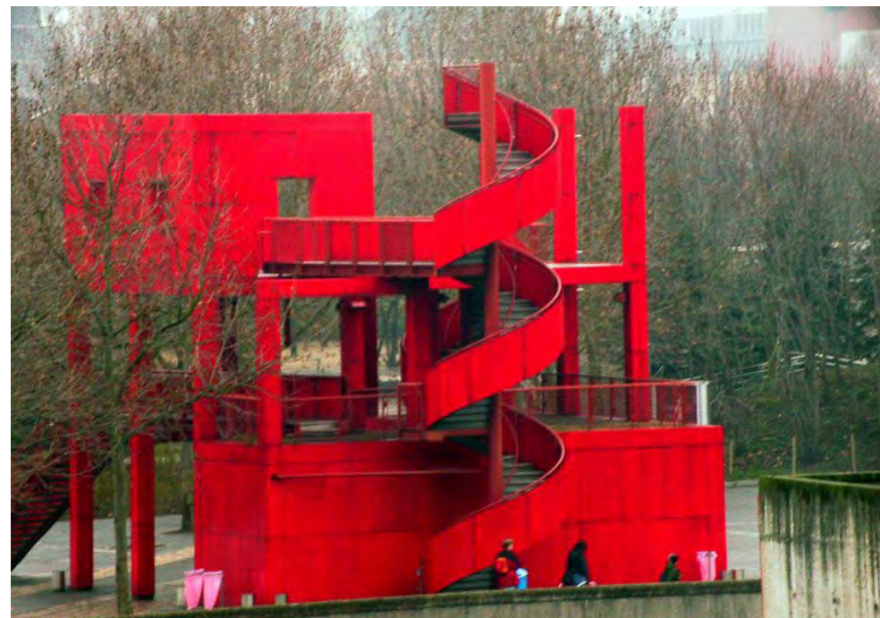
composition of stairs leading at the different levels of the building
