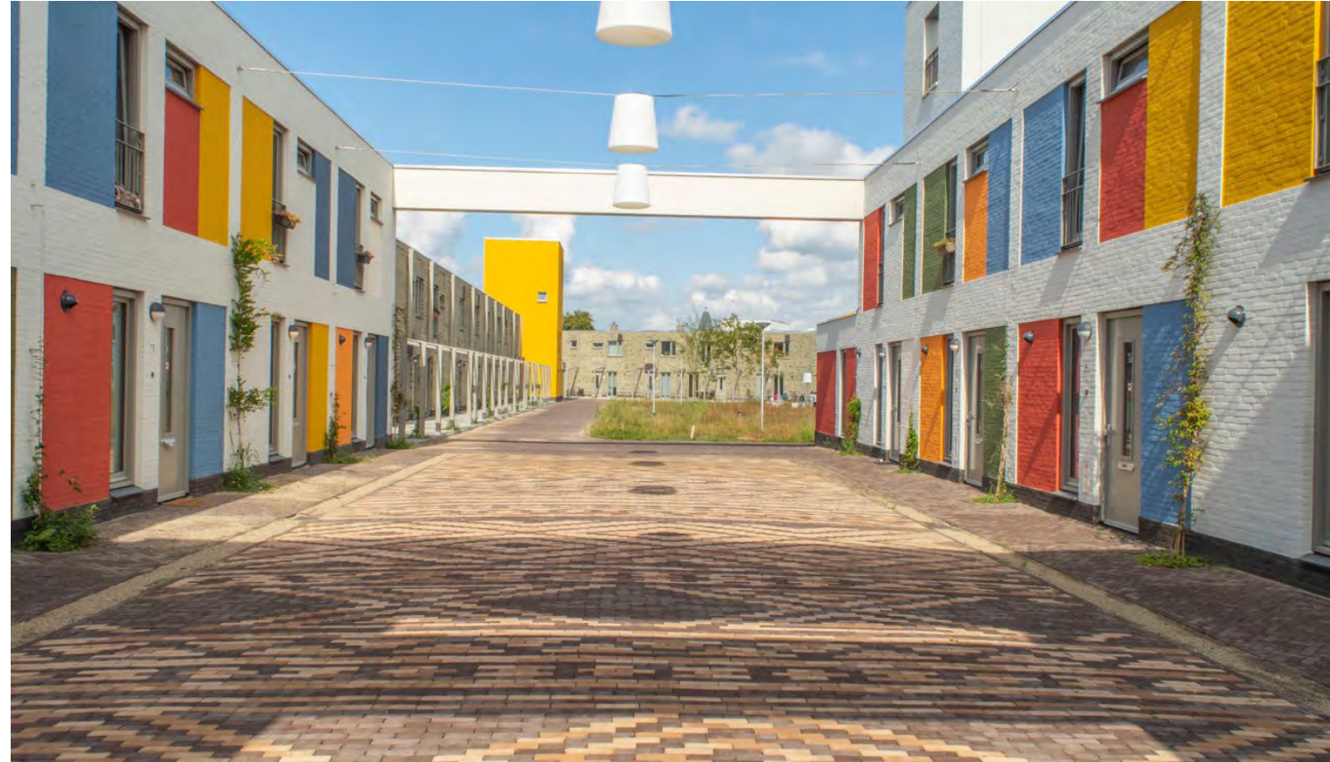
the area between the bridge and the market can be underlined by a special pavement
